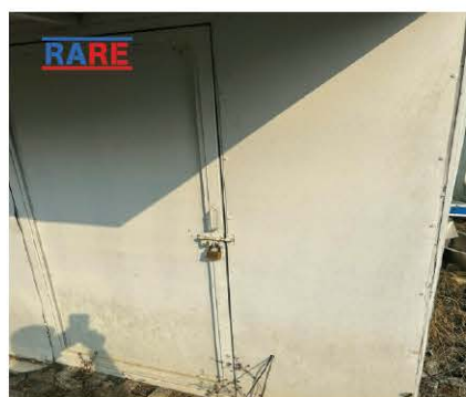
Sample construction in 1/2025 (after 5 years)
