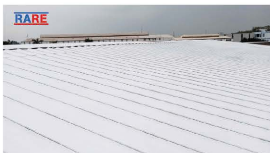
The roof surface is painted with RARE radiative cooling paint
