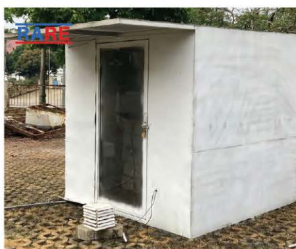
Sample construction in 2019
