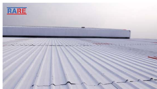
The roof surface is painted with RARE radiative cooling paint
