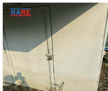
Sample construction in 1/2025 (after 5 years)
