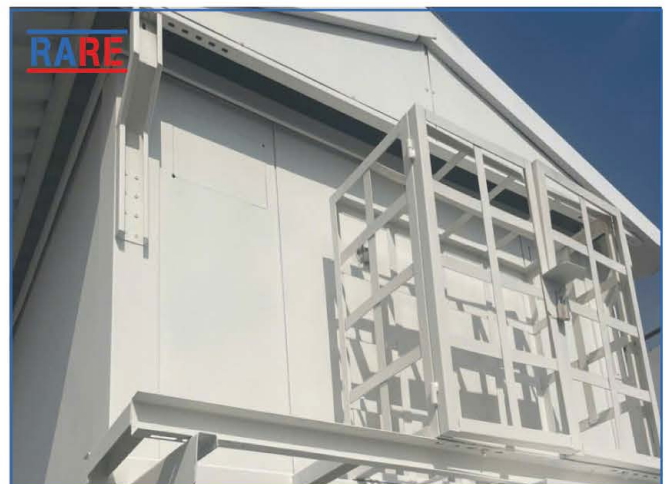
Coating for BTS Stations
