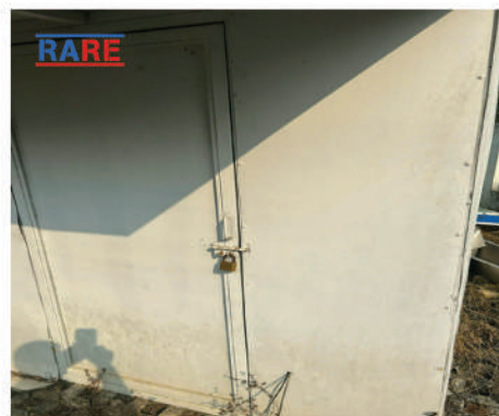
Sample construction in 1/2025 (after 5 years)
