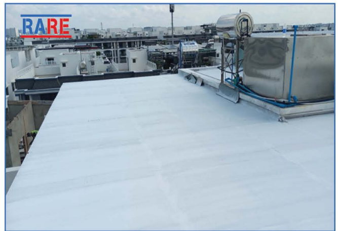
Coating for Walls and Rooftops
