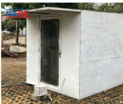
Sample construction in 2019
