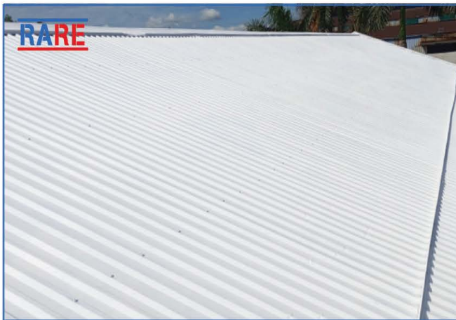
Coating for Metal Roofs
