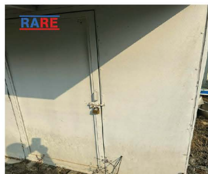
Sample construction in 1/2025 (after 5 years)
